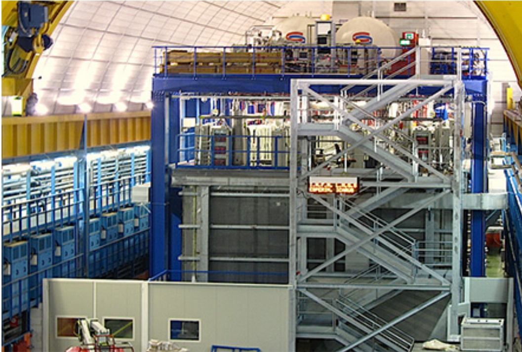
Figure 1. The ICARUS T600 plant in the Northern side of the Hall B at LNGS. Ladders to access the intermediate and the top levels are visible in the front together with the 3 m high wall that separates the T600 area from the rest of Hall B. Cabinets with the readout electronics are visible at the intermediate level. At the top level, the two 30 m 3 cryogenic storage tanks and some additional electronic equipments (HV supply, PMT electronics, trigger system, etc.) are also visible. Most of the cryogenic equipment (nitrogen and argon pumps, cryo-coolers, etc.) is located on the rear side of the T600, at the Northern end of the Hall B.
