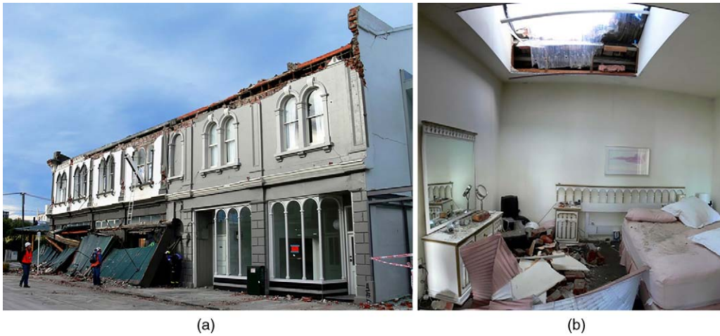
Figure 1. Examples of parapet failures during the 2010/2011 Canterbury earthquakes: (a) URM parapet that has collapsed onto the street frontage; (b) URM parapet that has collapsed into the building interior.
