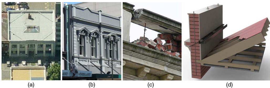
Figure 13. Other types of parapet interventions: (a) corner steel bar connection; (b) lightweight polystyrene replica; (c) insertion of vertical steel bars; (d) design scheme of the vertical bars.
