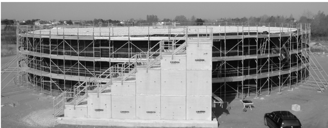
Figure 35. Trial embankment on completion.
